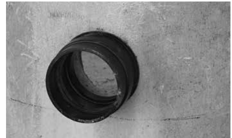
6. Installed EZ-Bell Adapter Coupling ready for service.
