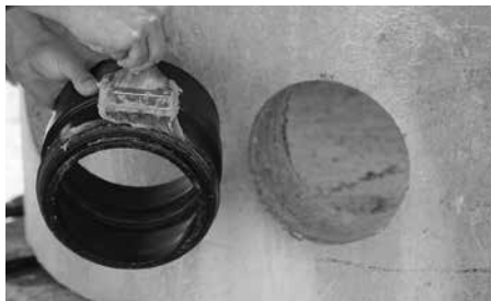
4. Lubricate the gasket of the EZ-Bell Adapter Coupling.
