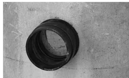
6. Installed Corebell Adapter Coupling ready for service.
