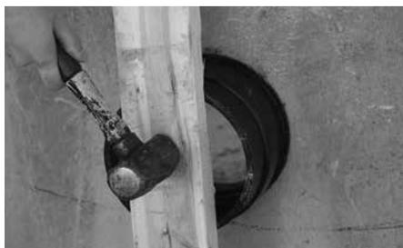
5. Use a flat block of wood and hammer to knock and seat the Corebell Adapter Coupling into place.
