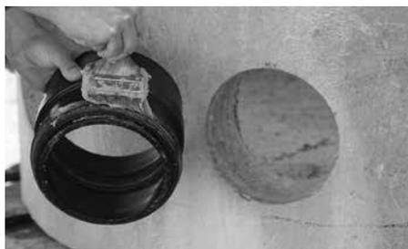
4. Lubricate the gasket of the Corebell Adapter Coupling.
