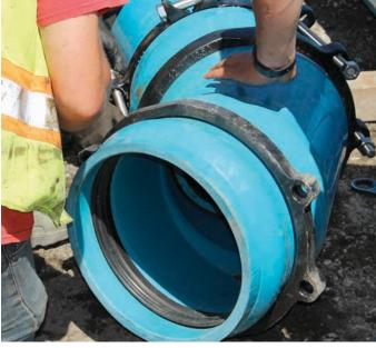
Fabricated Pressure Fittings are manufactured from AWWA C900 pipe 100mm to 1200mm (4" to 48").
