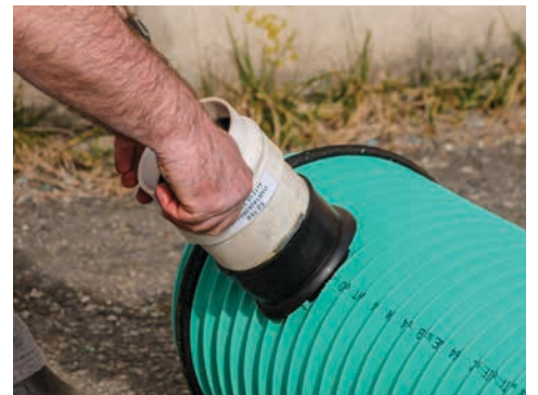
4. Insert lateral connection into gasket
