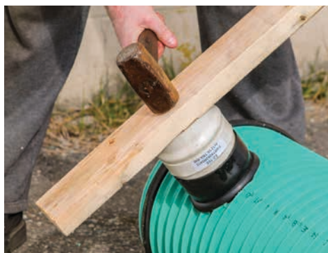
5. Use a block of wood or a similar substitute to set the lateral connection
