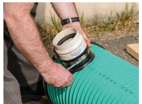
6. Tighten the stainless steel clamp to conclude the installation
