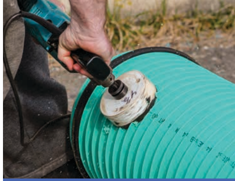
1. Core hole (run drill in reverse)
