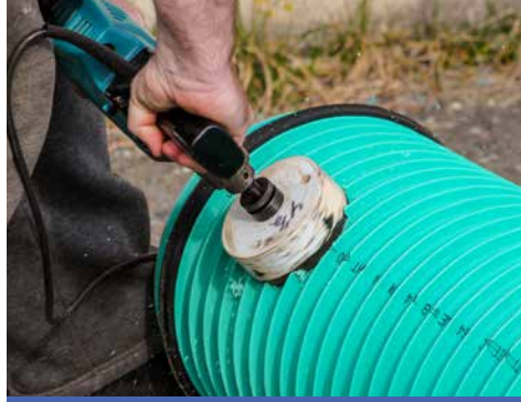
1. Core hole (run drill in reverse)
