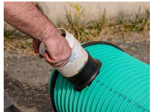
4. Insert lateral connection into gasket
