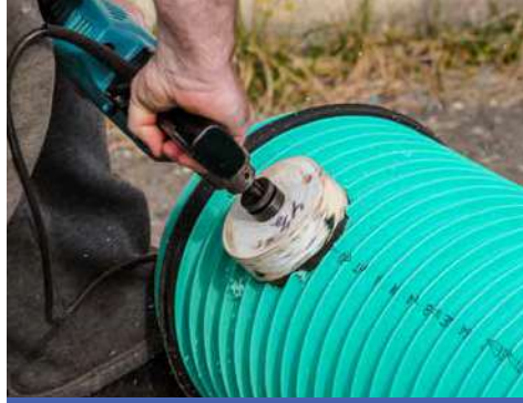
1. Core hole (run drill in reverse)
