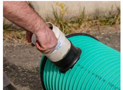
4. Insert lateral connection into gasket
