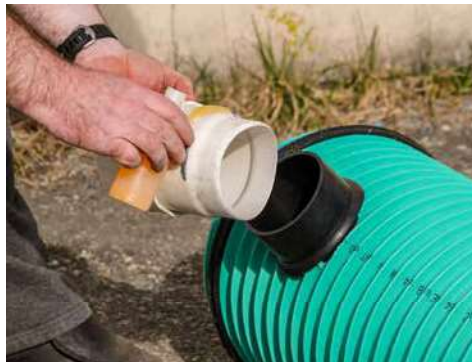
3. Lubricate the spigot end of the lateral connection
