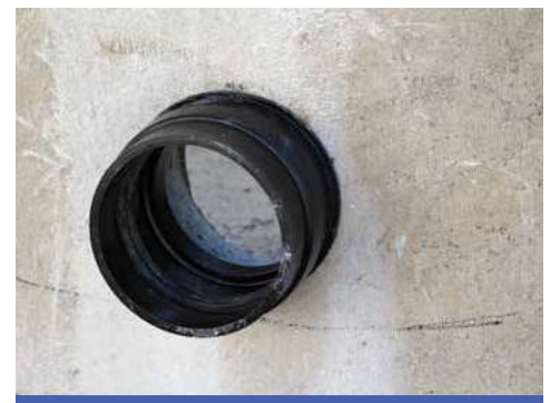
6. Installed Corebell Adapter Coupling ready for service
