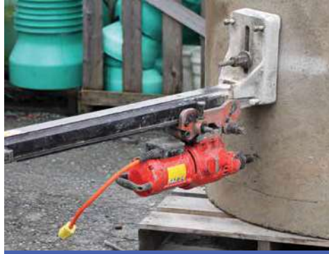
1. Mount saw jig to manhole
