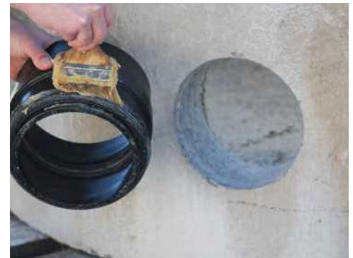
4. Lubricate the gasket of the Corebell Adapter Coupling
