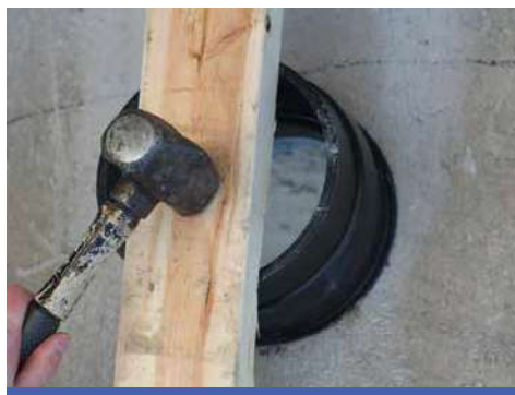
5. Use a flat block of wood and hammer to knock and seat the Corebell Adapter Coupling into place
