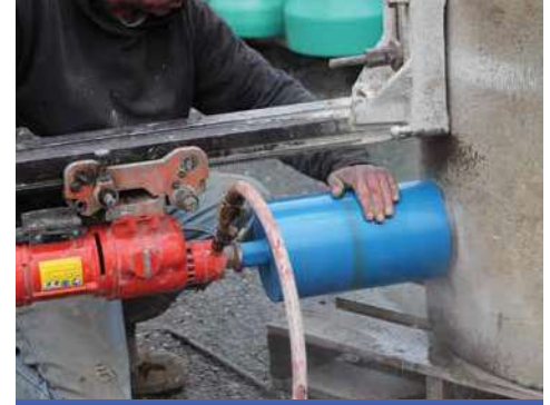
2. Drill/Core manhole
